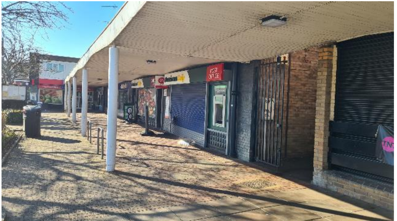
Figure 11: Avon Drive shops
