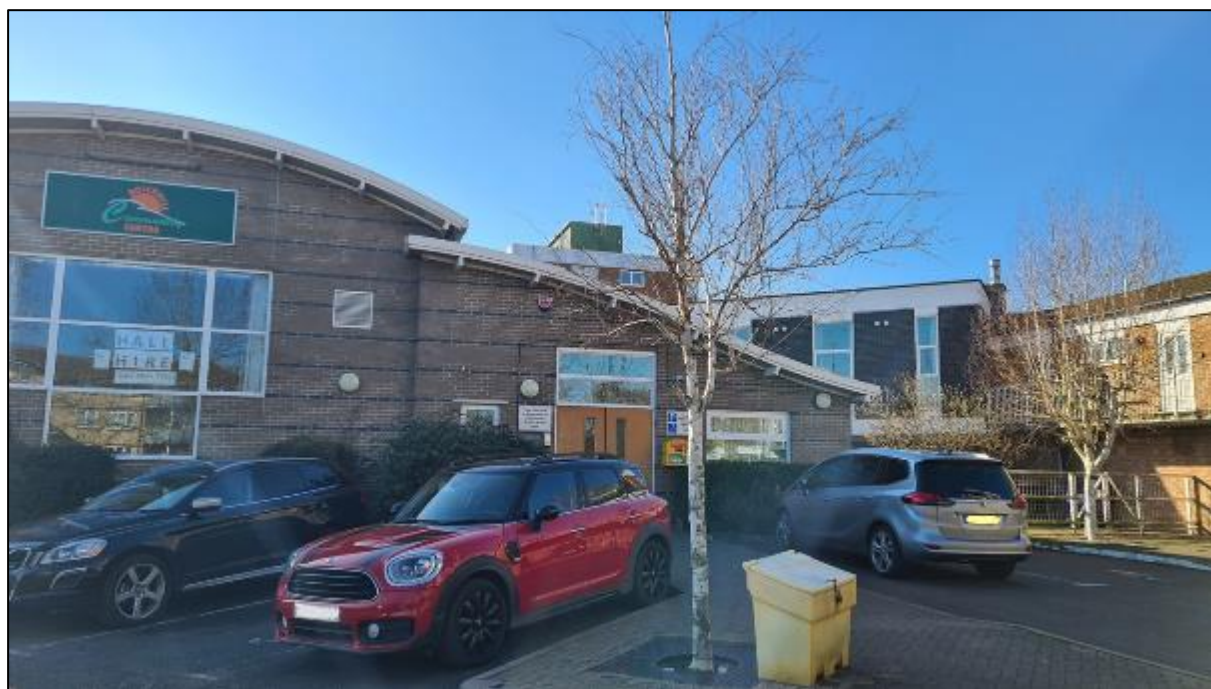
Figure 7: Brickhill Community Centre
